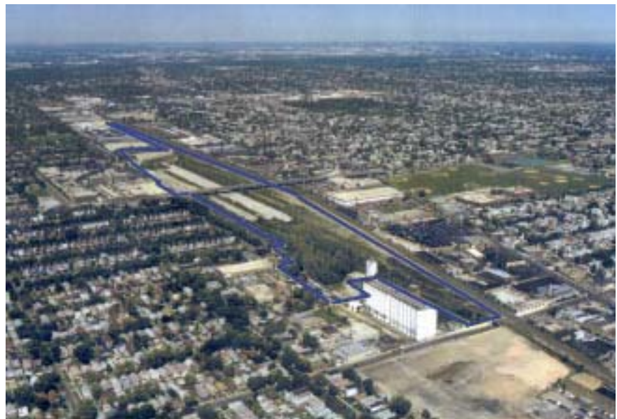
Aerial view of the Galewood Yards
